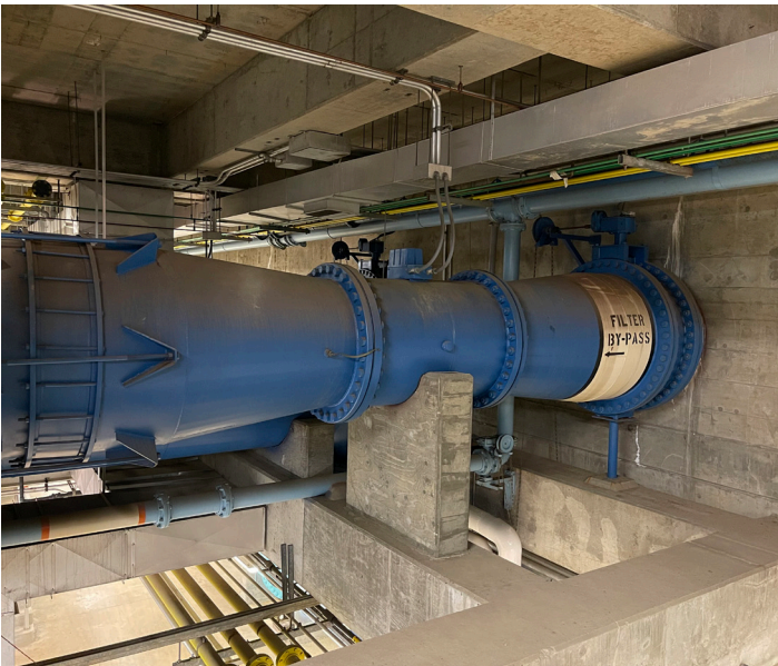
A 48" butterfly valve installed in a filter bypass line was not a good solution for handling the dirty media because of the disc in the center of the flow path.
