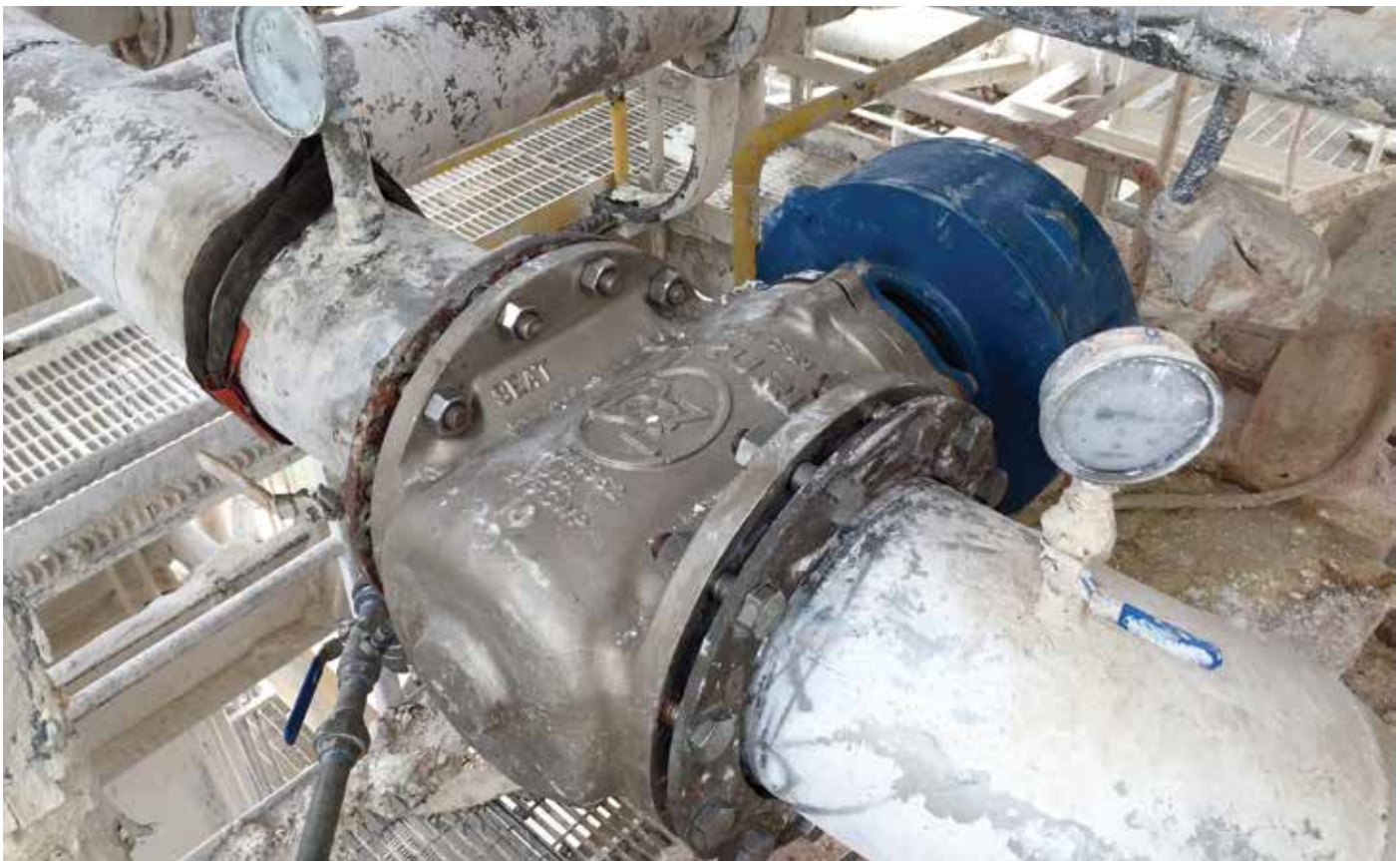
DeZURIK PEC Eccentric Plug Valve in pulp mill green liquor isolation
