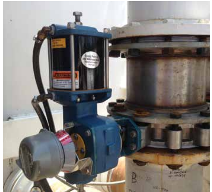
DeZURIK High Performance Butterfly Valves are ideally suited for a wide variety of services including water, steam, liquor and other corrosive liquids and gases.
