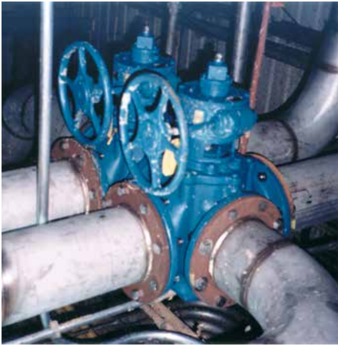
DeZURIK's 3-Way Tapered Plug Valves are designed for throttling and diverting applications in refiner stock control applications.
