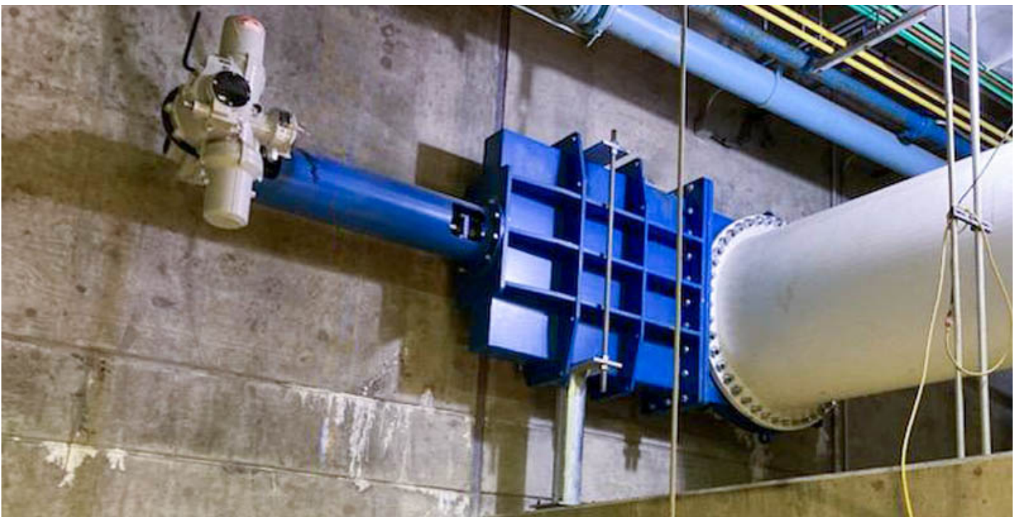
The Hilton Bonneted Knife Gate Valve includes gate guides, a drain port, and actuator support to accommodate the horizontal mounting position.
