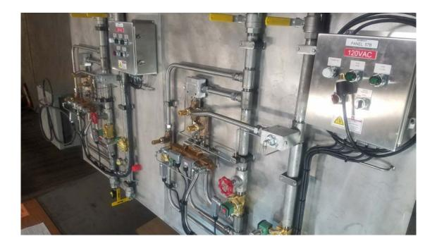
DeZURIK's low pressure hydraulic accumulator systems are an on-demand system that operates automatically and supplies pressurized fluid to the pressure header. Plant monitoring of the accumulator system is available either hardwired or with a communication module.
