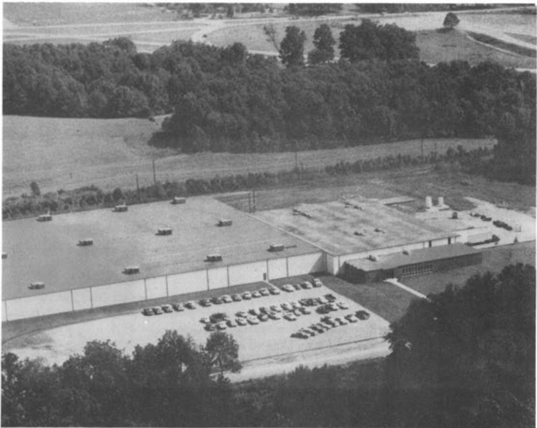
McMinnville, TN Plant 1965.
