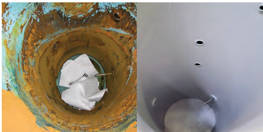
FIG. 5. Reservoir tank of hydrodesulfurization unit before and after maintenance.
