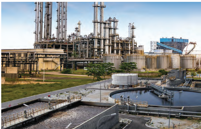
FIG. 1. Wastewater recycle and reuse at HPI/CPI facilities is becoming a trend. Treated wastewater can be recycled for use onsite or in other beneficial areas such as cooling tower makeup, service water, boiler feedwater and, in some cases, irrigation.
