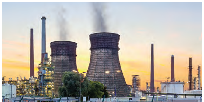
FIG. 4. Cooling tower operation and maintenance costs can be high. Water management companies can recommend strategies for facilitating delivery of consistent, high-quality makeup water, and can develop cooling tower blowdown discharge and reuse solutions.
