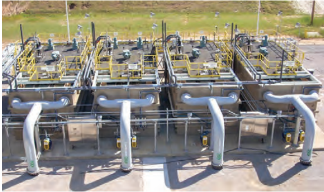
FIG. 5. A proprietary, high-rate softening technology lowers the raw water footprint. The system combines microsand-ballasted coagulation, flocculation and lamella settling to treat raw water and wastewater.
