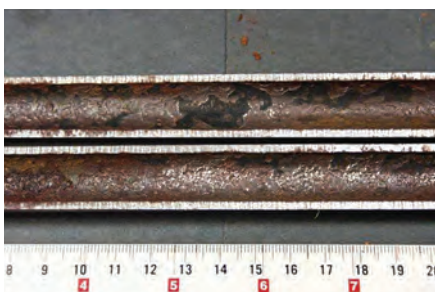
FIG. 2. A large under-deposit corrosion pit (with deposit removed) in a stainless-steel heat exchanger tube.
