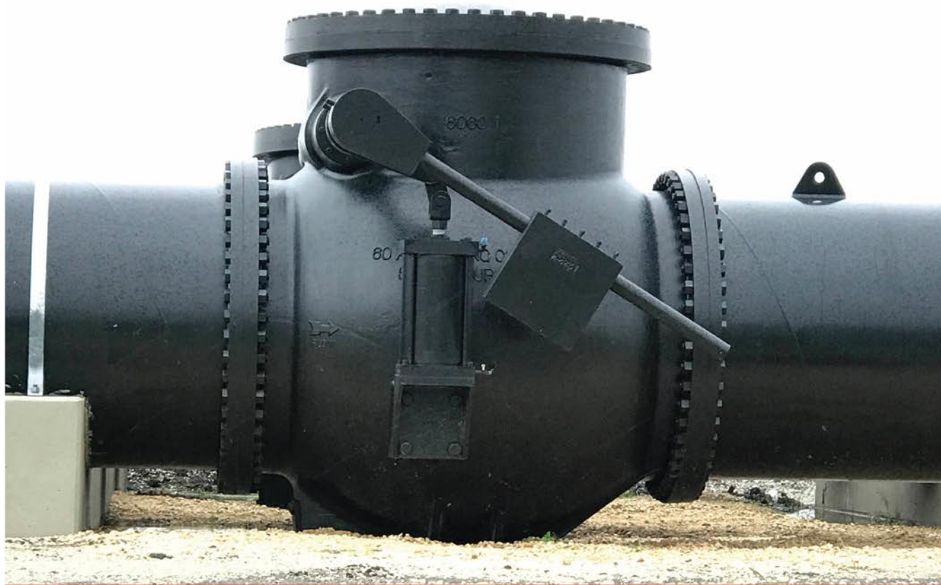
60-inch swing check valve for critical backflow prevention.
